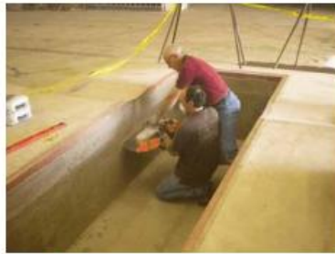
Cut Wall for hoses
