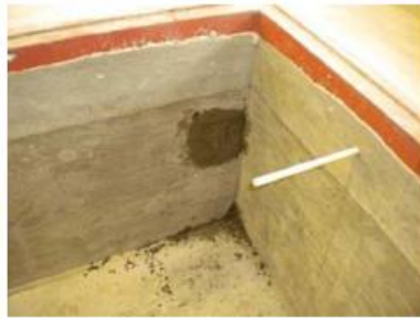
Sealed Concrete Gaps
