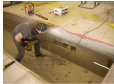
Chipped concrete for hoses
